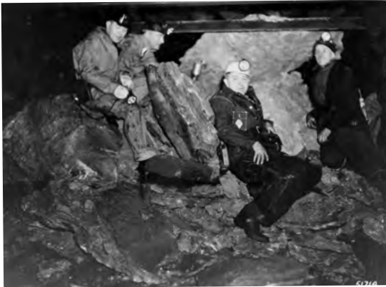
Showing typical roof falls along entries following explosion.
