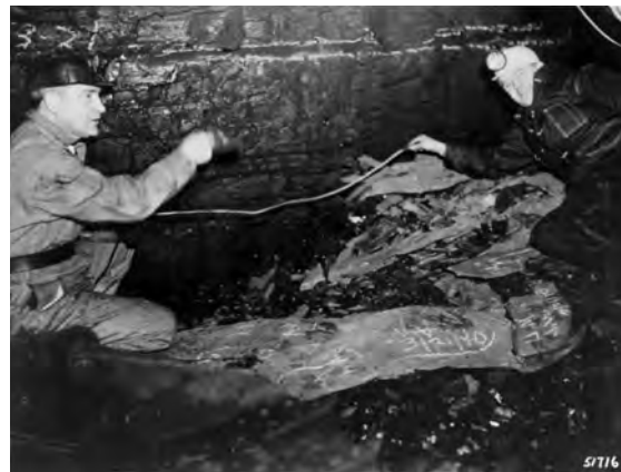
Showing Shot firing cable stretched out from a hole.
