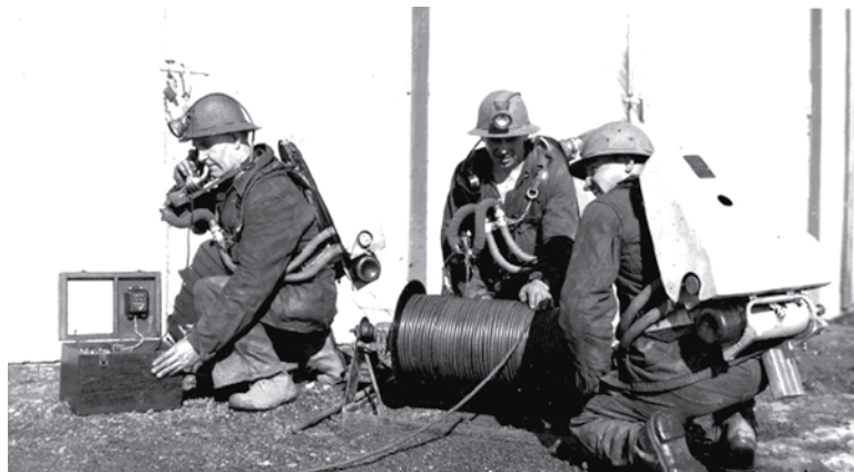
Figure 1, 1940s sound-powered mine rescue communication system
