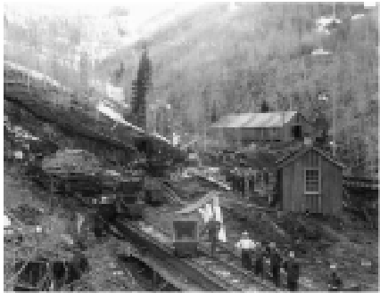
The devastation after the explosion outside on Mine No. 4, where the explosion originated
