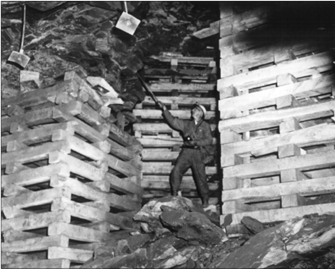
Miner scaling loose roof after a fall—notice the hanging bolts
