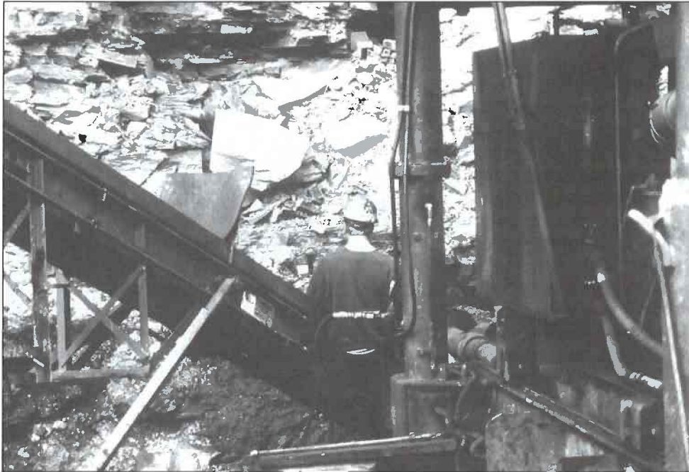
Independent contractor workers augering into highwall
