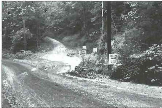
At left, straddle berms constructed from soft material serve to quickly slow the momentum of a runaway truck. The ramps are angled to permit the driver to guide his truck into them with a minimum of steering.
