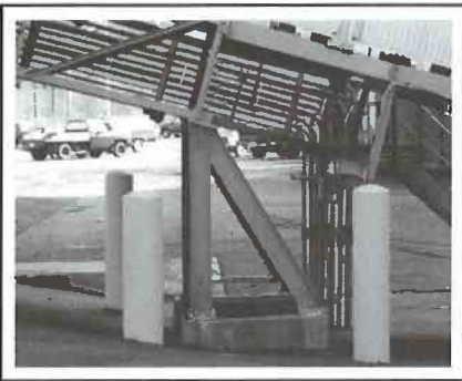
Photo 3 above, shows guards to protect supports from accidental strikage. Photo 4 at right, a fixed guarded ladder. Photo 5 below right, installation of stairway to check fluid levels in pumps.
