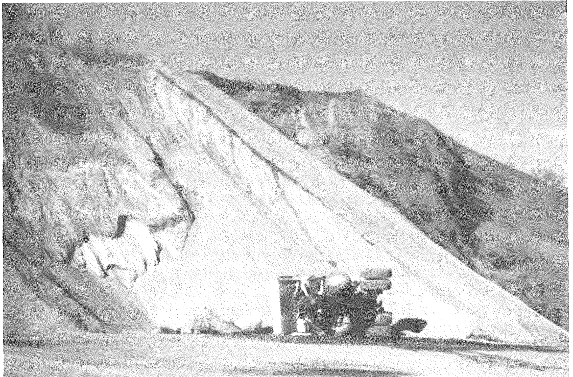
Figure 1.—Accident due to collapse of edge of pile.
