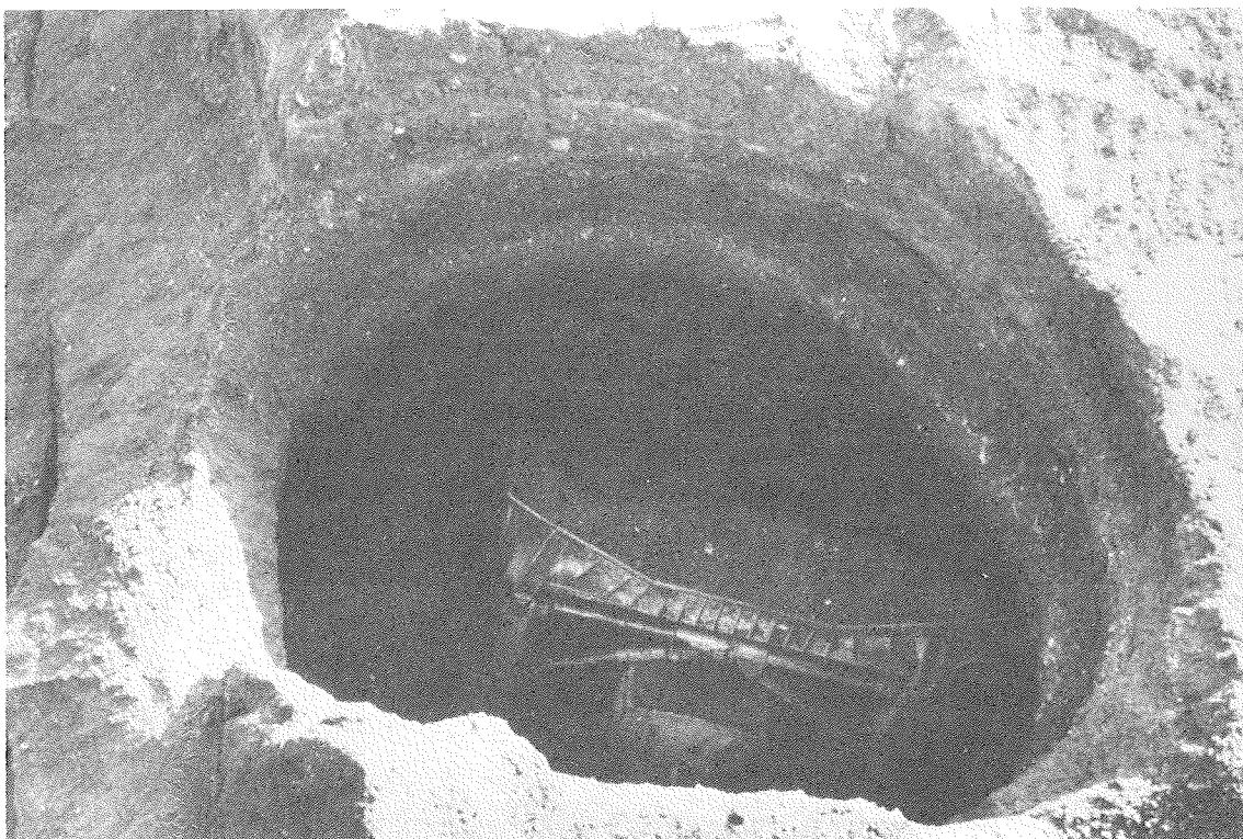
Figure 2.—Dozer in drawhole.
