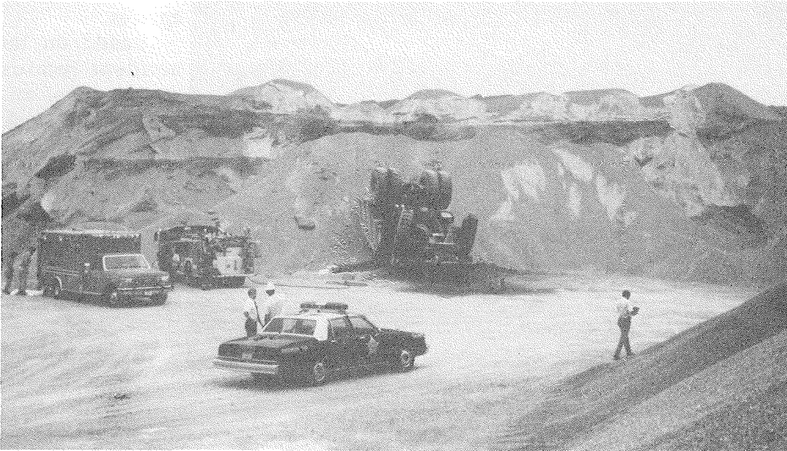
Figure 1. —Accident caused by collapse of stockpile edge while truck was in process of dumping over side of pile.
