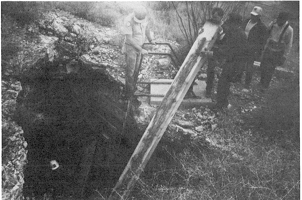
Hauling timber Jeff Dexter, manager of Kartchner Caverns State Park, and other Arizona Parks Department employees lower a 16-foot 10 x 12 timber down the sink hole for miners to install in the caverns opening, seen at left of the photo.
