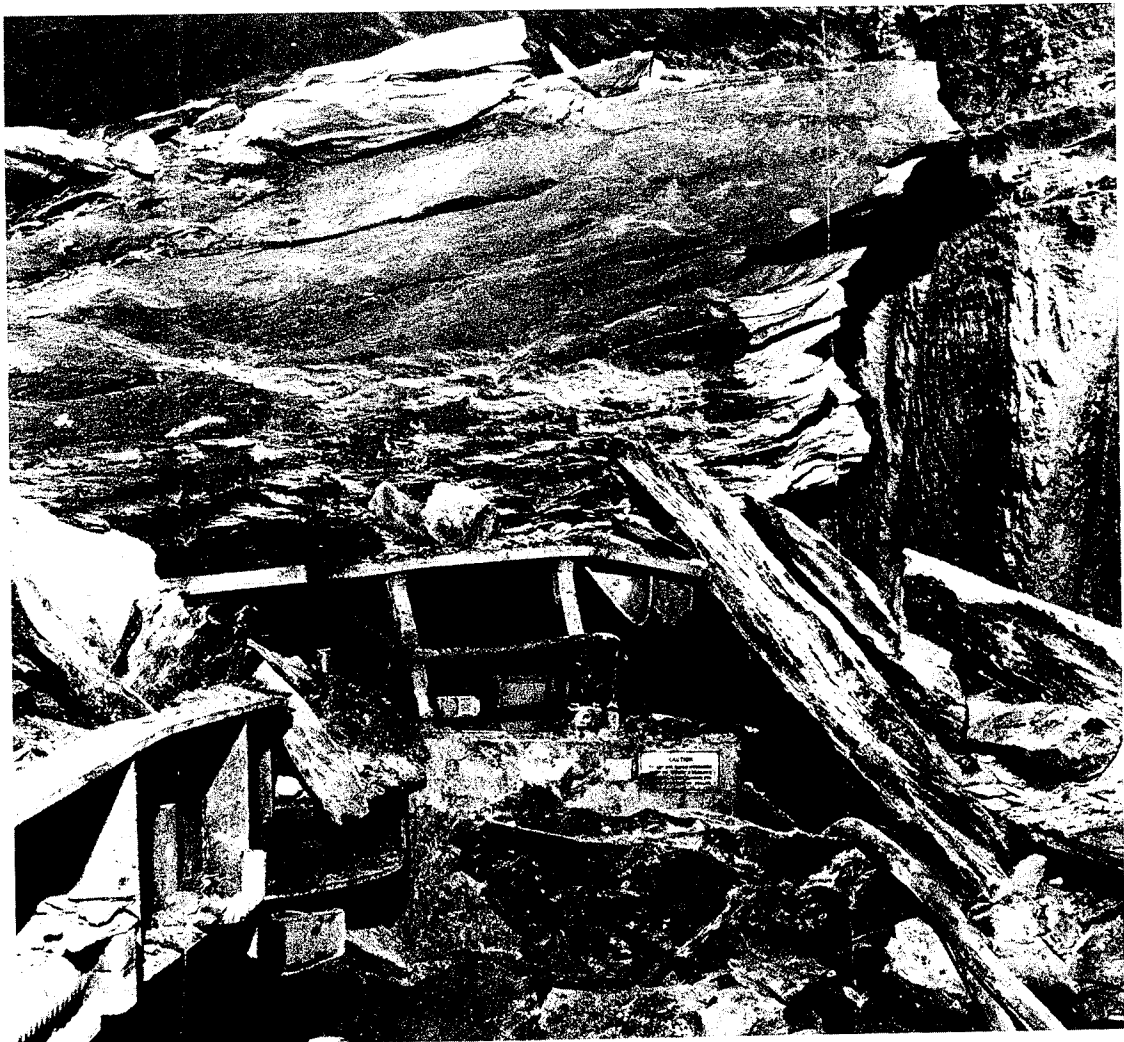
Canopy saved the miner in this roof fall
