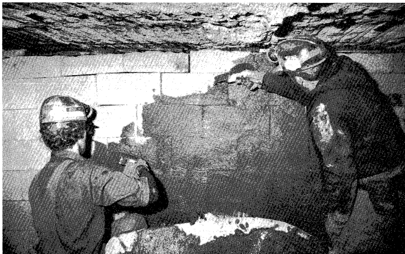
Mine workers brush-applying modified mortar on a concrete block stopping.
