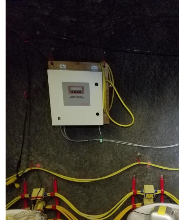
Real-time SF6 concentration monitor (Maximum concentration-1000 ppm)
