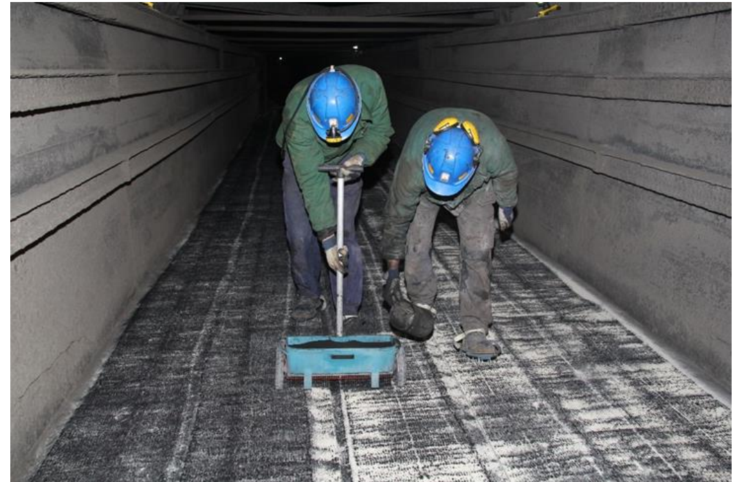
Applying 75 kg of coal dust on top of rock dust
