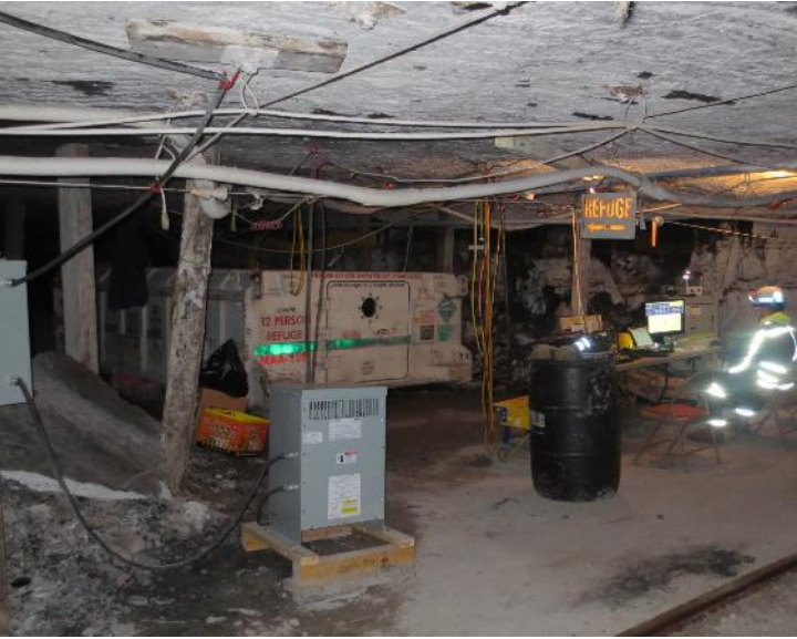
Carbon-dioxide-based Cooling System
