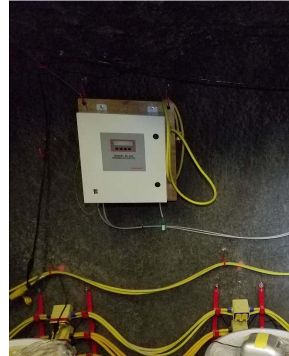
Real-time SF 6 concentration monitor (Maximum concentration-1000 ppm)
