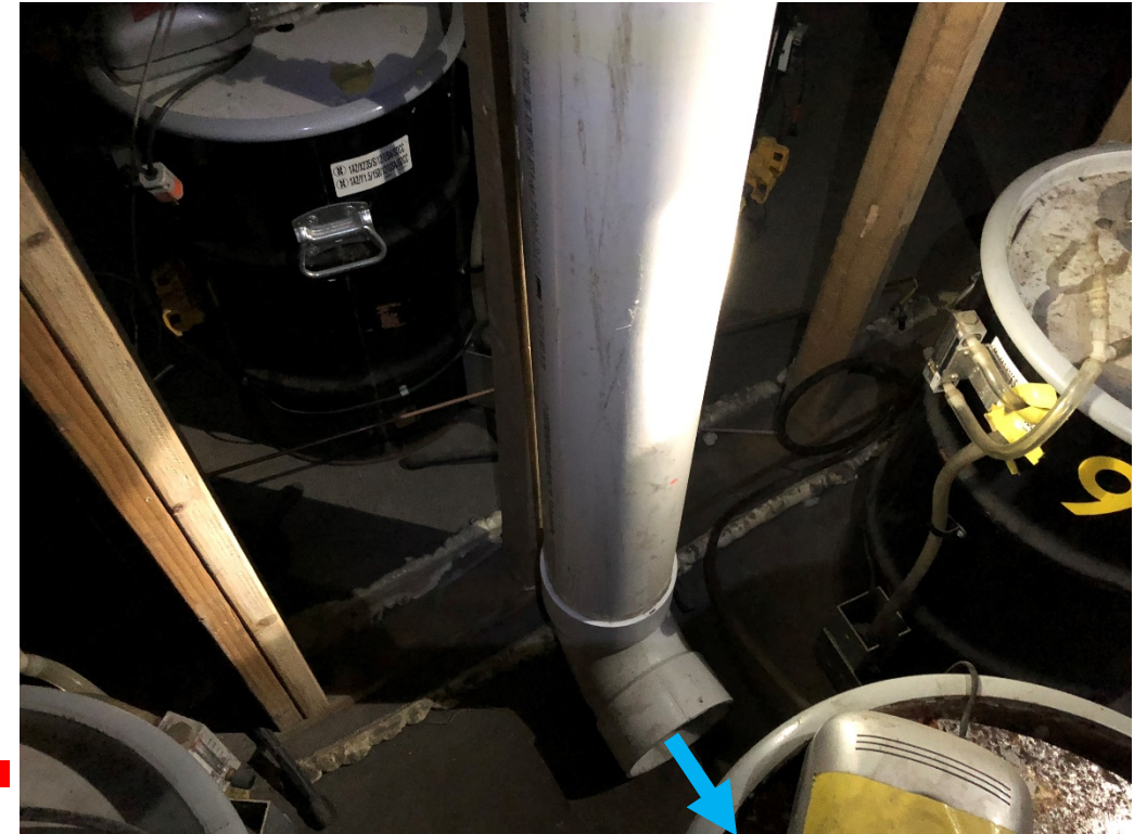
Air inlet for MVSC #8
