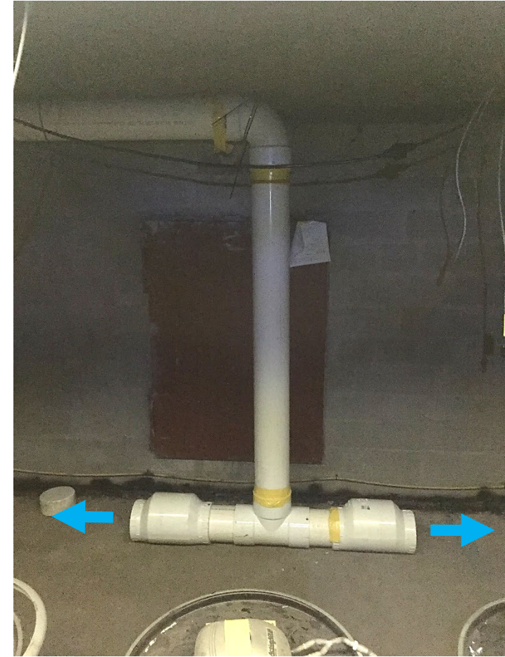
Air inlet for MVSC #2, 3, 12
