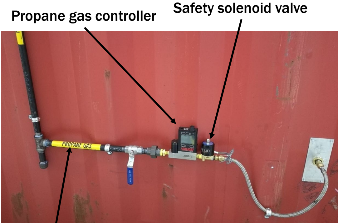
Propane gas line
