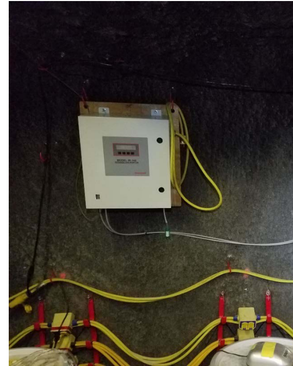
Real-time SF 6 concentration monitor (Maximum concentration–1000 ppm)
