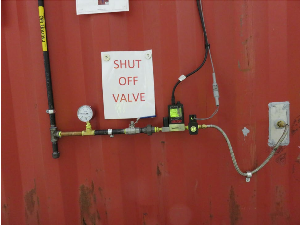
Propane Delivery Lines
