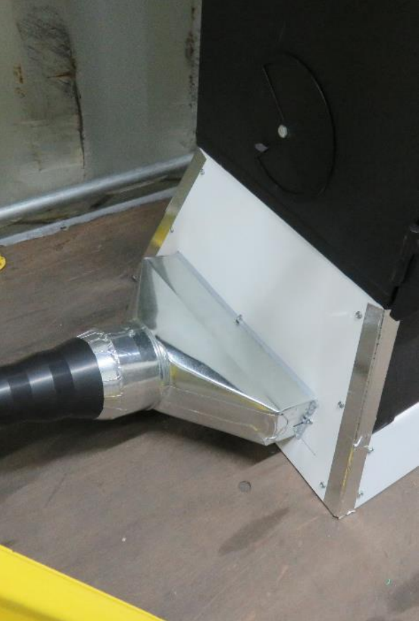
Combustion Air Inlet
