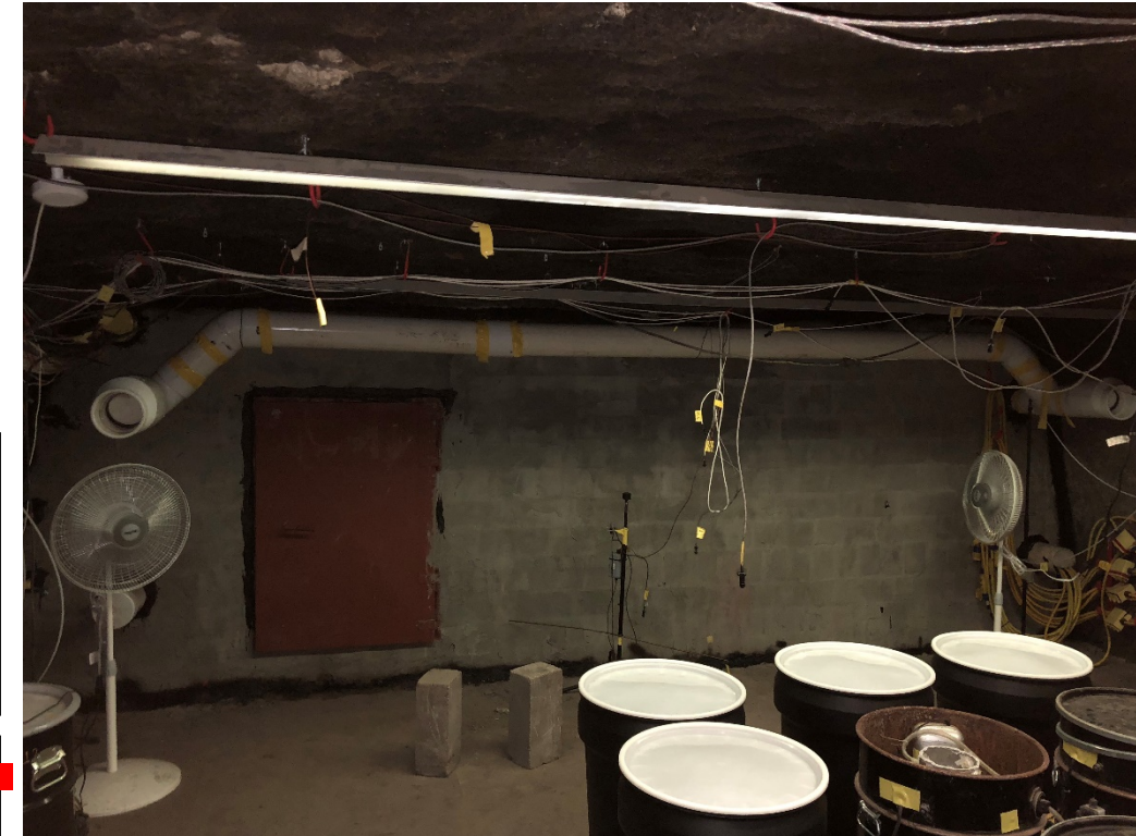
Y-shaped air outlet for VSC #3, 4
