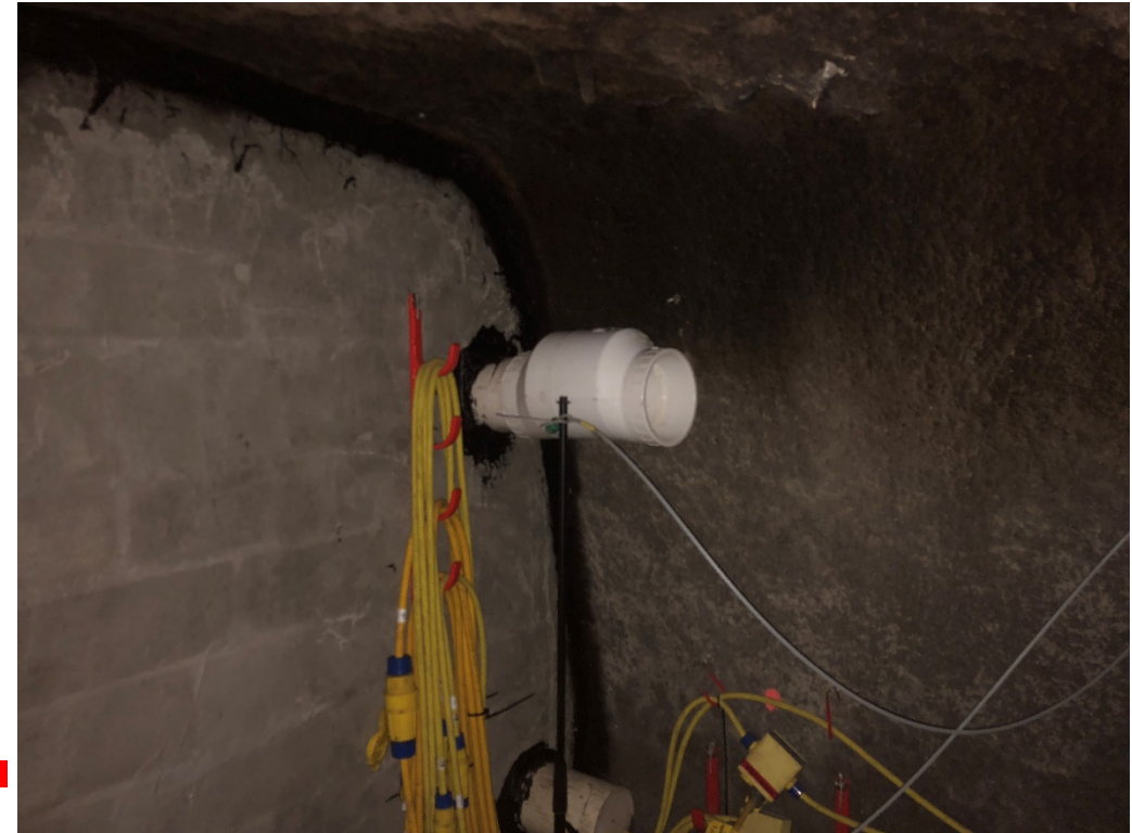
Air outlet for VSC #1, 2, 5, 6, 7, 8, 9, 10, 11, 12
