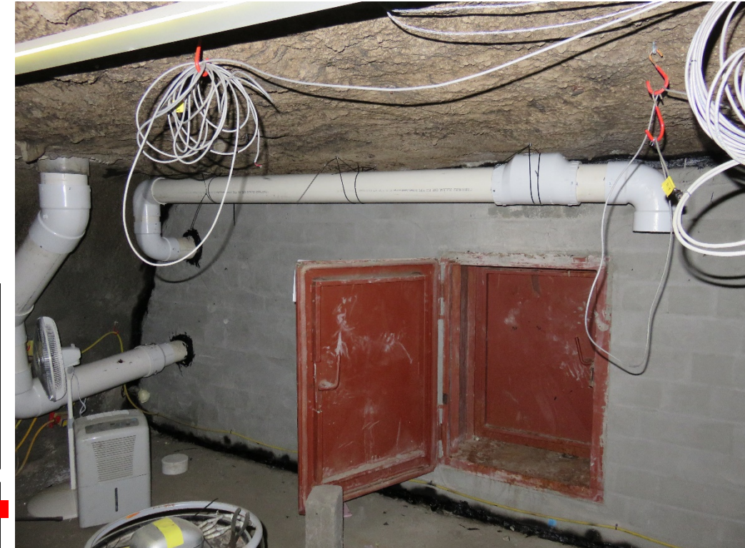
Air inlet for VSC #1
