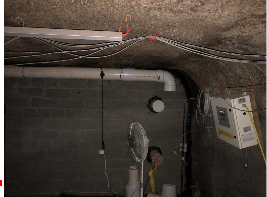
Air inlet for VSC #4, 5
