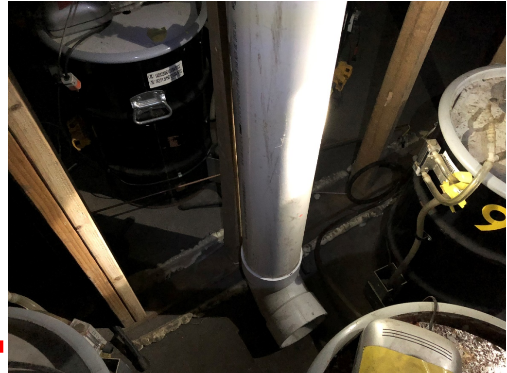
Air inlet for VSC #8
