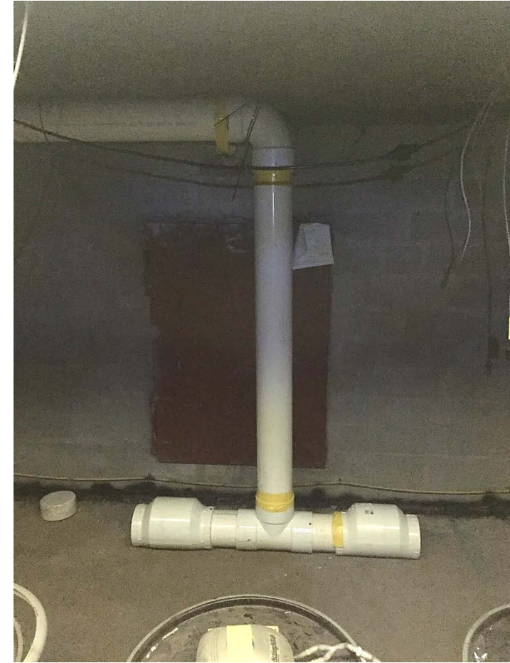
Air inlet for VSC #2, 3, 12
