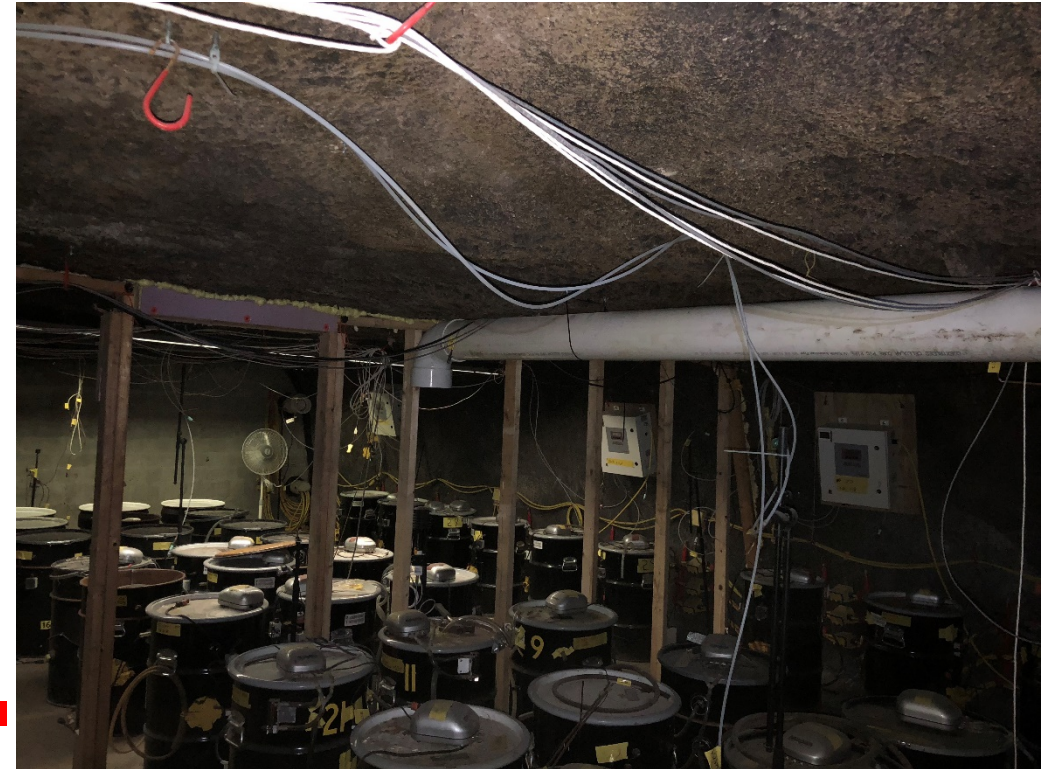
Air inlet for VSC #7, 10, 11
