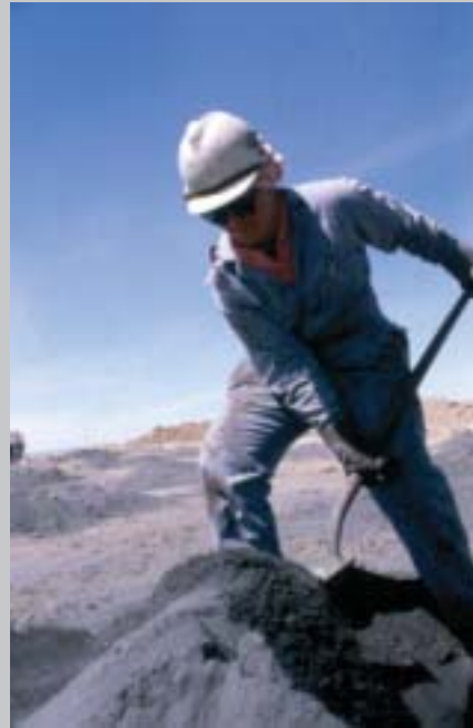
Make recommendations on using the proper tools and equipment
